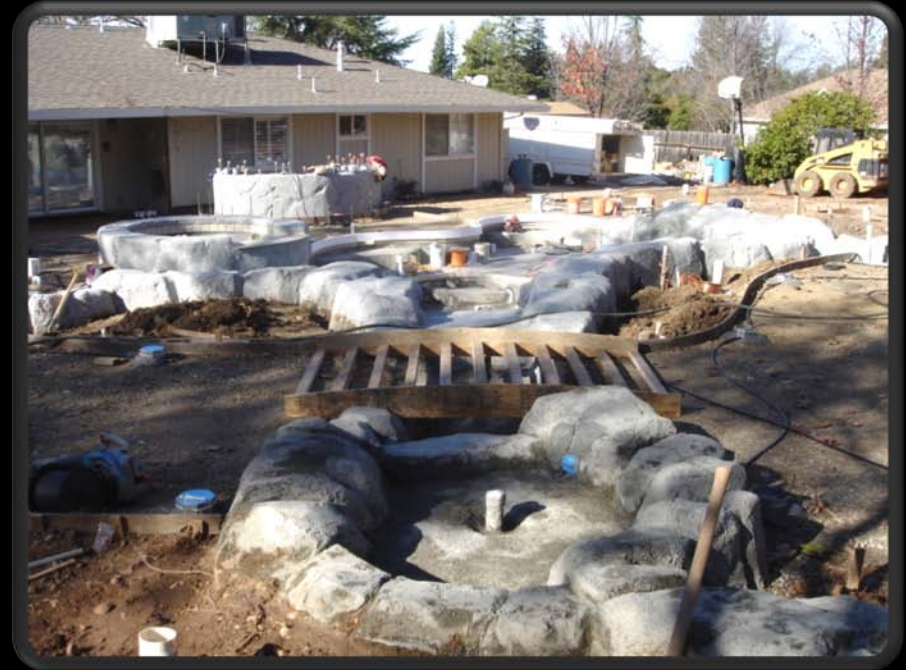
CONCRETE DECK FORMING
